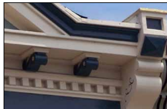
Above: Brackets and Cornice
